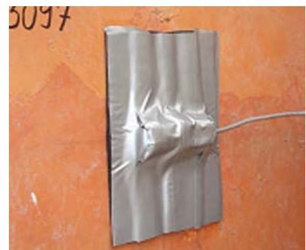
Figure 3.3 Further thermal protection by duct tape
