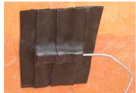
Figure 3.2 Initial thermal protection by insulation tape
